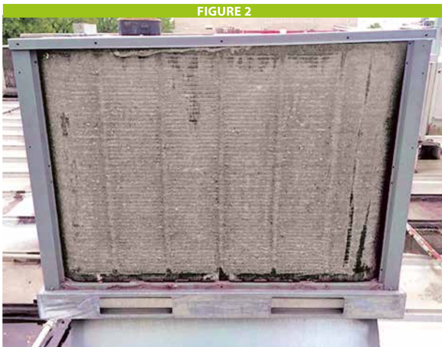
FIGURE 2 Condenseur excessivement sale
